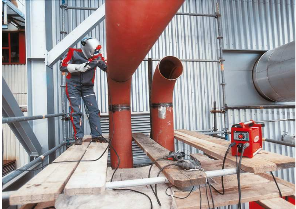
Fig. 30 Welding of pipe by method MMA
