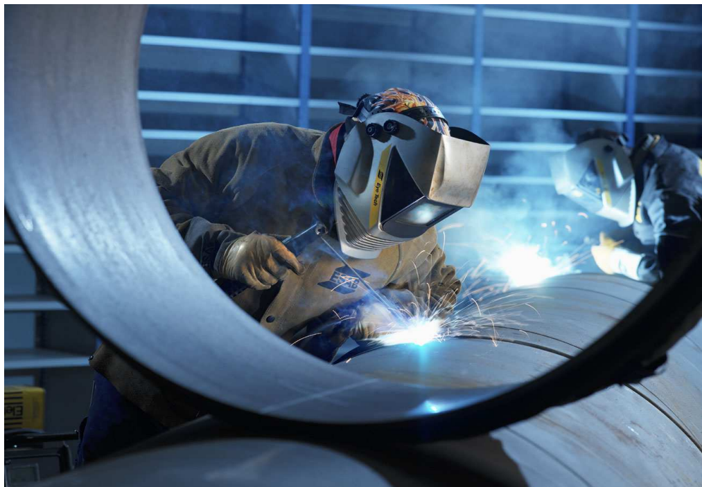
Fig. 29 Welding of rolled steel by method MMA
