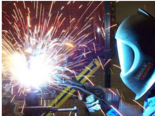
Fig. 13 Demonstration of manual welding
