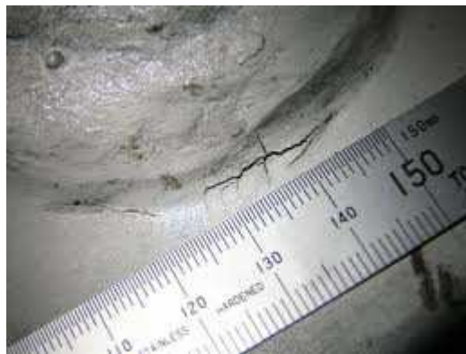
Fig. 44 Magnetic inspection of welds
