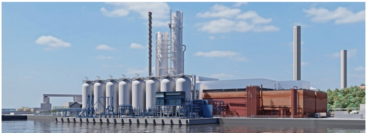
Figure 16: BECCS plant in Stockholm, Sweden. Photo by Beccs Stockholm 2 .
