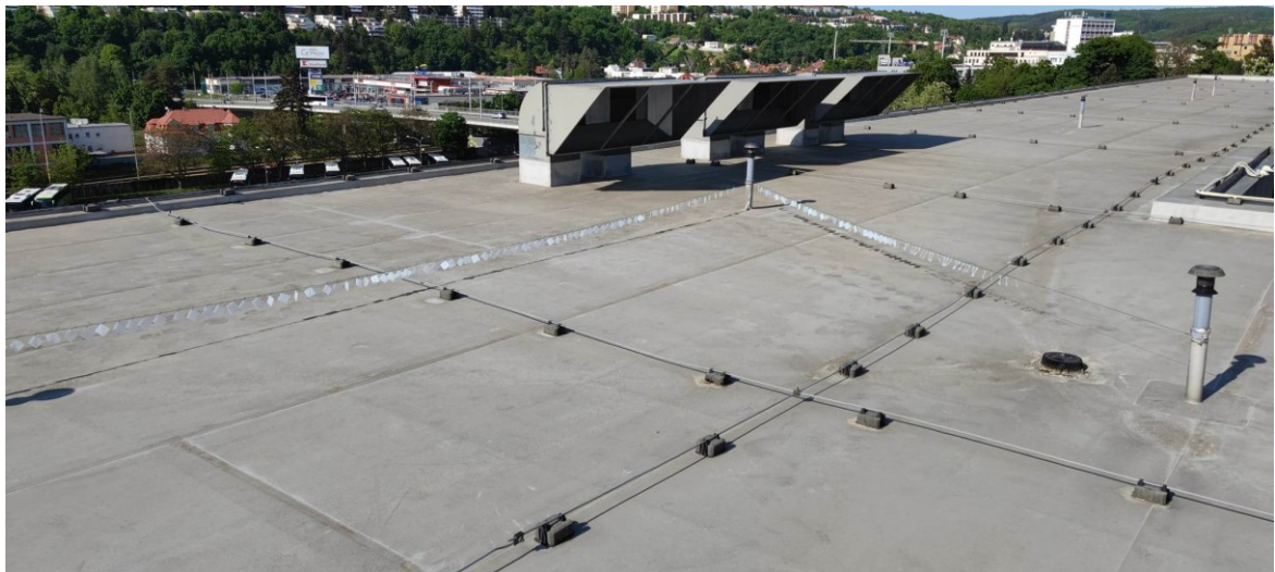
Figure 12 Samples on the roof at the day of the installation
