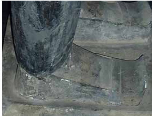
Fig. 38. Shoe with a stiffening hem [14]
